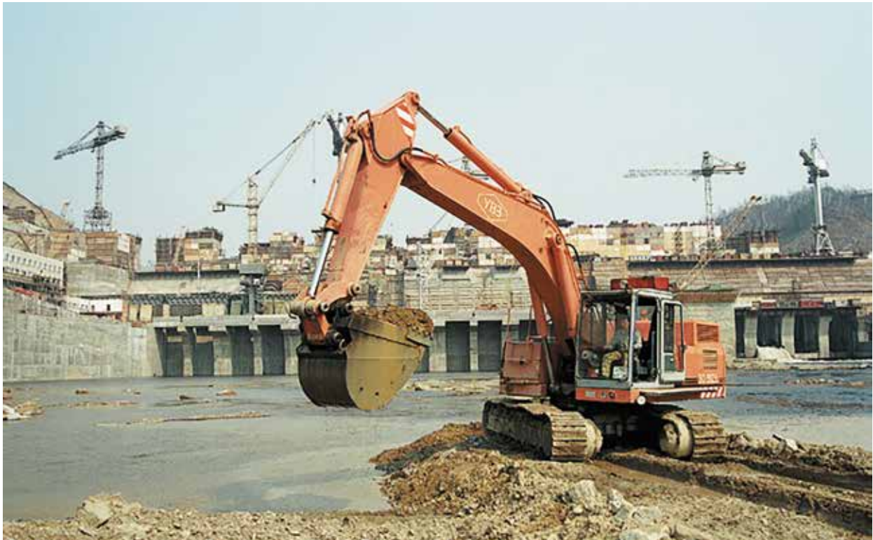
Construction of Bureyskaya Dam by WWF–Russia
