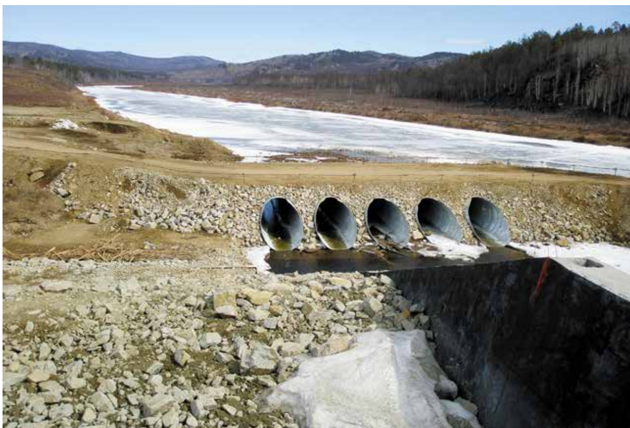
The Amazar pulp mill dam, the first reservoir financed and built by the Chinese in the Russian part of the Amur basin by Igor Shkradyuk
